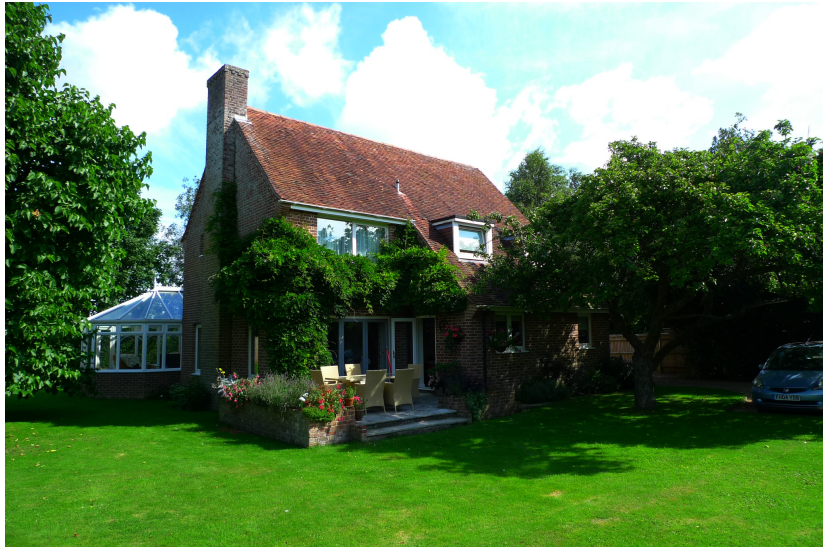
Photograph of house as existing
