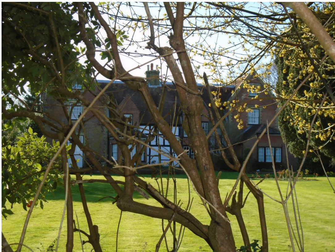
Figure 3. View of rear elevation from the recreation ground car park.
