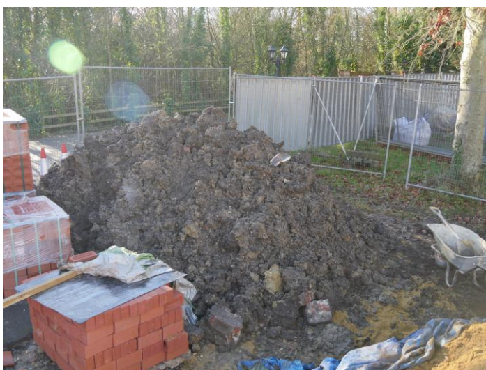
Photo 1 – Contaminated soil – stored at the side of the drive ready for collection
