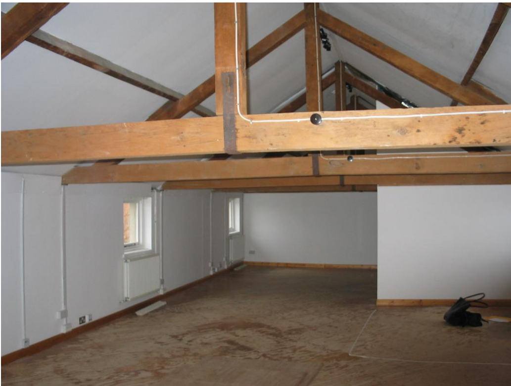
Interior of second floor - looking east
