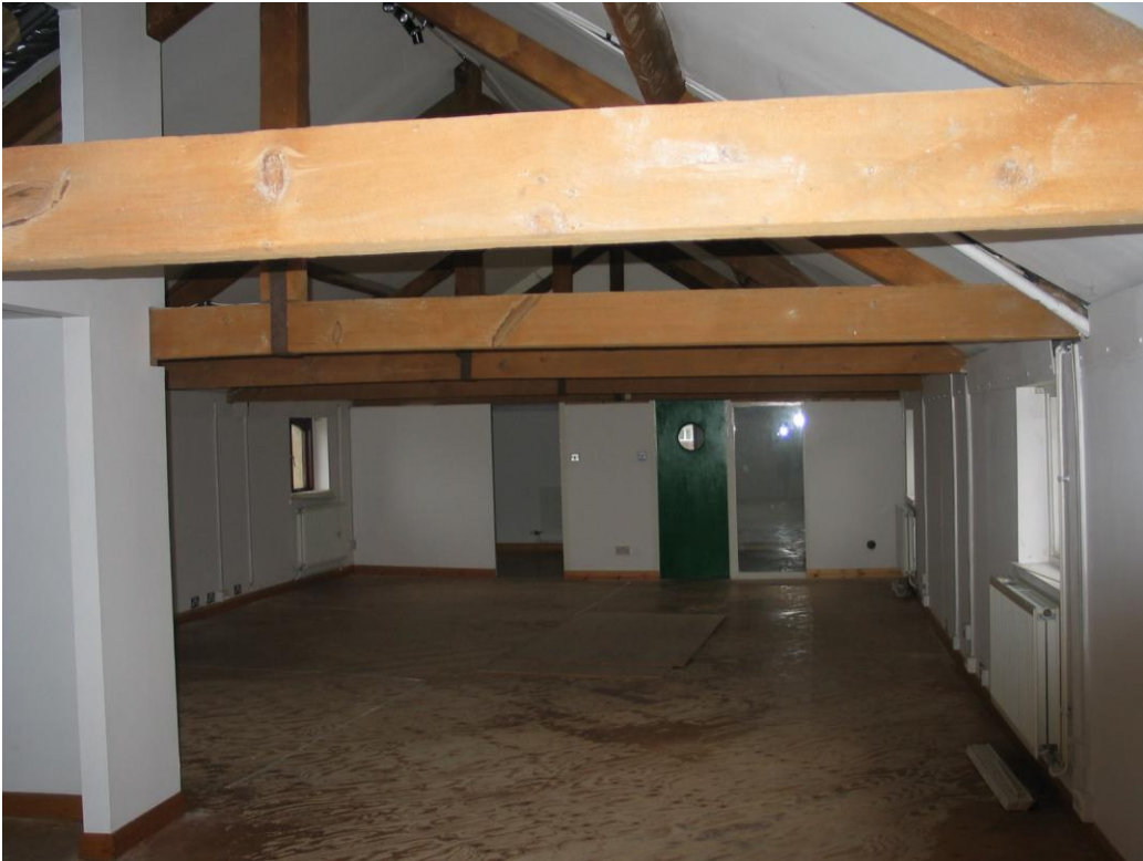
Interior of second floor of Malt House – looking west
