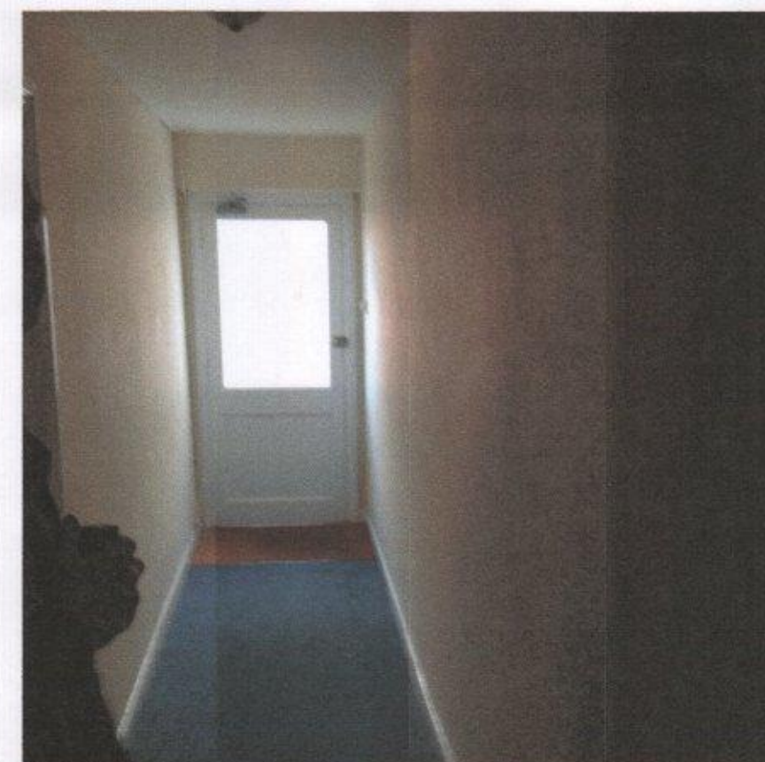
Common Hall Way Facing South
