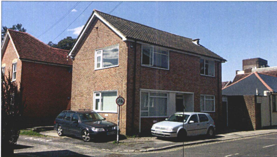
Entrance to existing ground floor office (proposed 2 bedroom flat)
