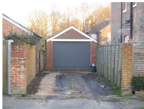
Fig 5 - View of existing drive and garage
