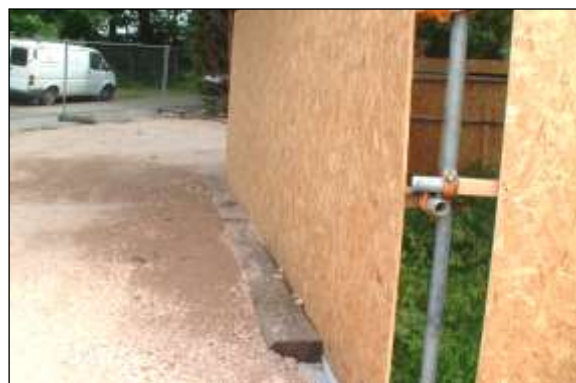
New surfacing image 5: Although this is only a temporary surface, railway sleepers pinned into the ground can be used to retain the edges of new surfacing.
