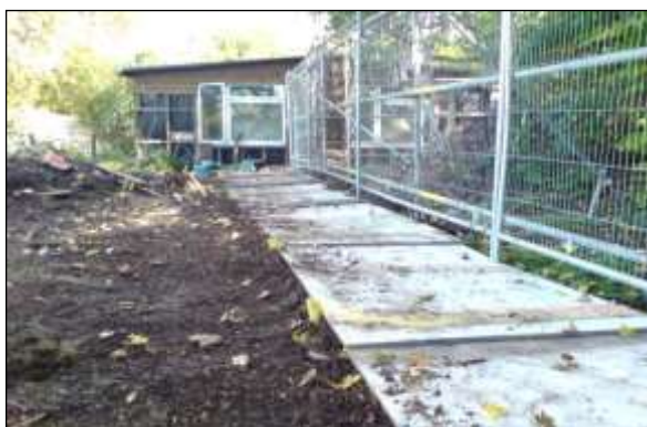
Ground protection image 1: Heavy-duty plywood set onto a compressible woodchip layer and pinned into position is suitable
