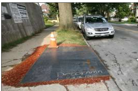
Ground protection image 8: Steel plates can be an effective way of temporarily reinforcing weak surfacing over a construction access during the development activity.
