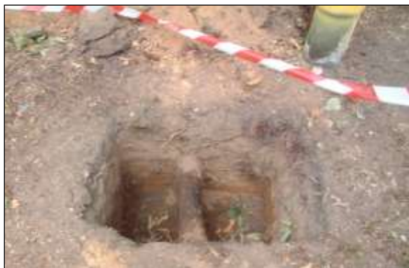
New structure image 1: Where posts are proposed close to trunks, it is essential to excavate 50–75cm deep to see if there are any significant roots in the way, with provision to move the post hole location if roots are found (note the post was finally installed to avoid this root).
