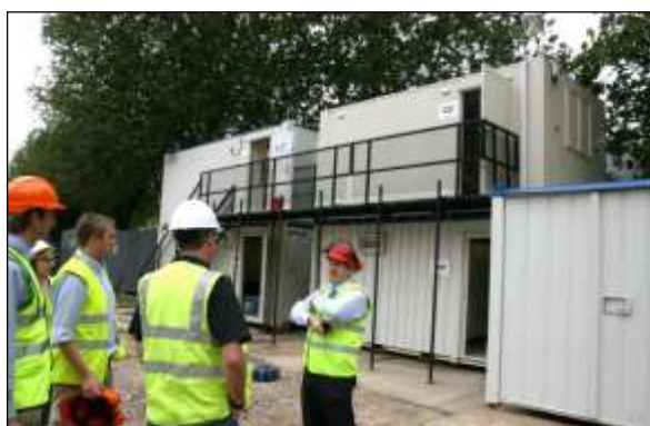
Ground protection image 7: A combination of retaining existing surfacing and using temporary construction cabin accommodation can be a very effective means of preventing damage to sensitive areas.
