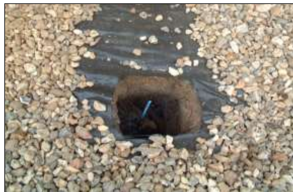
New structure image 2: Ground protection must be used to spread the load during excavation.
