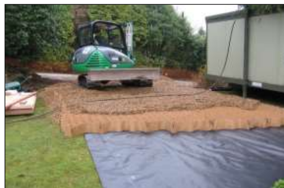
New surfacing image 3: The stone-filled cells spread the load of traffic and the geotextile membrane on the ground prevents migration of the stone into the soil profile.
