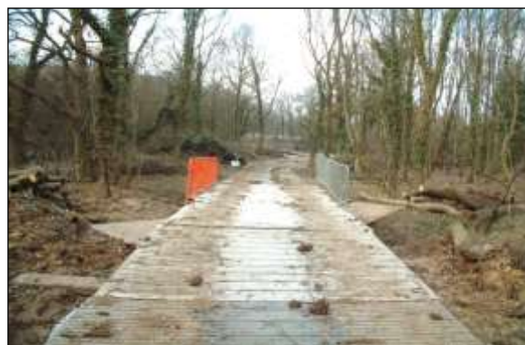
Ground protection image 6: Custom designed sectional tracks can be joined to support very heavy traffic use through sensitive areas.
