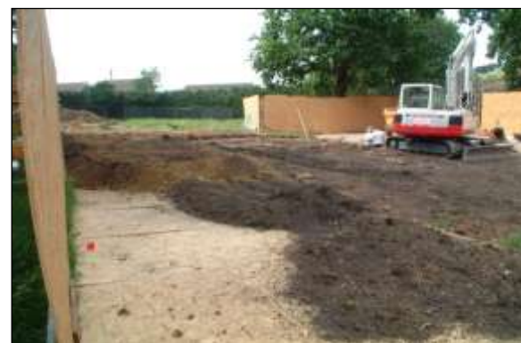
Ground protection image 2: Spreading soil excavated from footings is an effective way of buffering the plywood surface from
