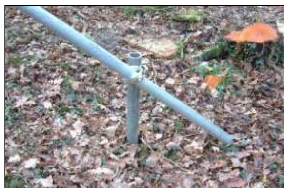
Fencing image 3: Close up of bracing detail, essential for increasing the stability of the vertical framework.
