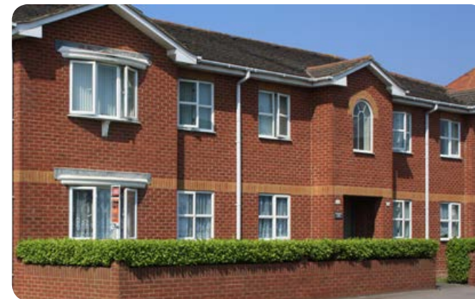
Example of a modern block of apartments along a main route through the island
