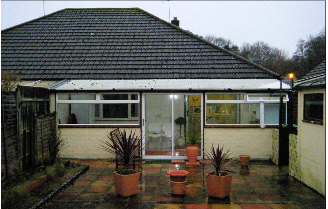
Rear of No. 2 showing conservatory
