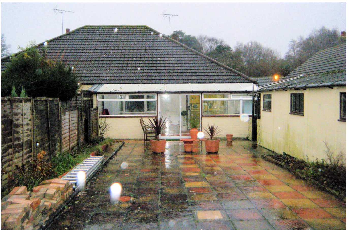
Rear of No. 2 showing conservatory and location of extension
