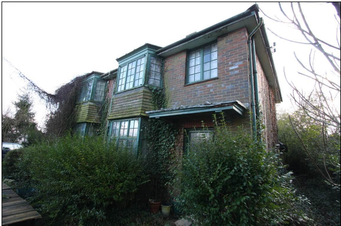
Photo 11 Manor Farm House is 2 semi-detached houses
