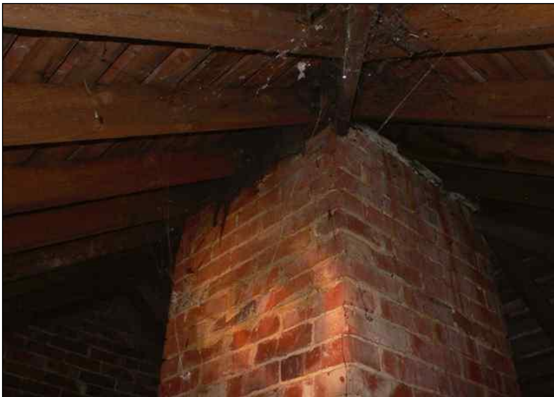
Photo14: Internal Chimney Structure
