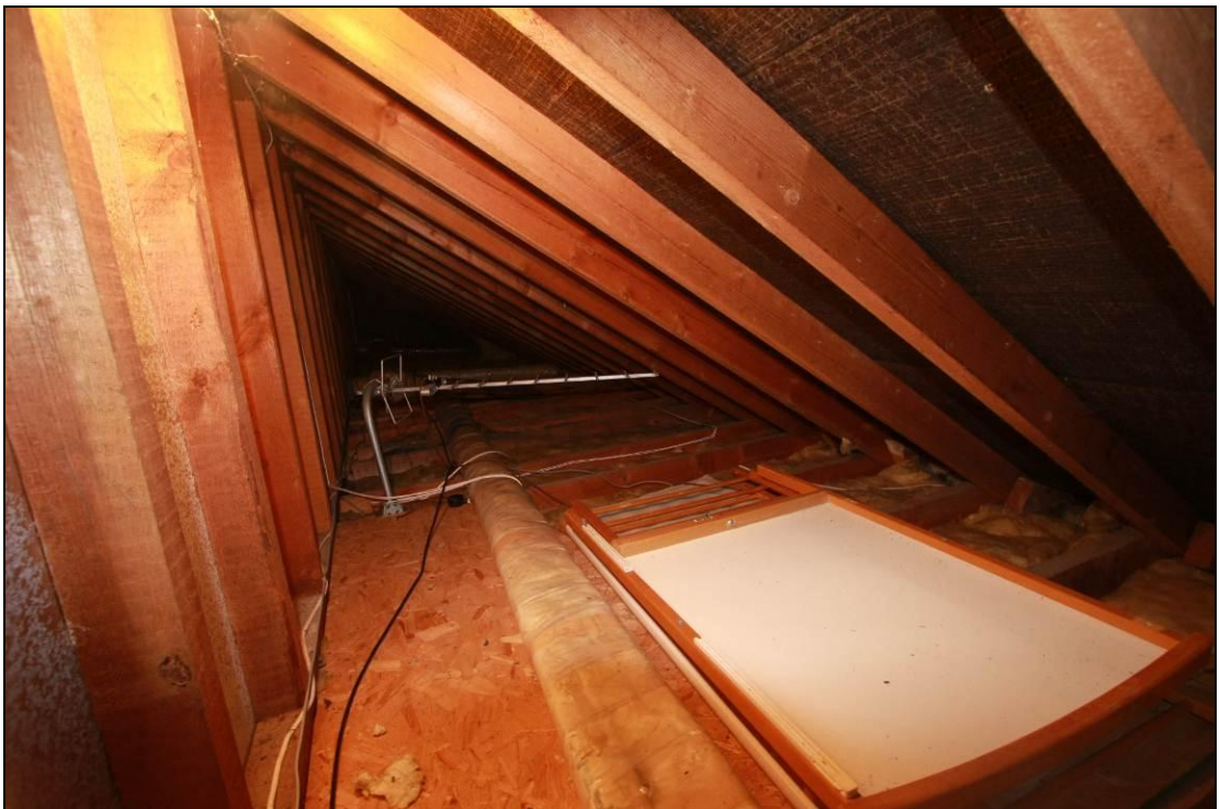
Photo 21: Internal Roof Voids in the converted roof space of the dwelling, used as storage with lighting and some boarding. No evidence of Bat use, extensive mouse droppings and two Wasps nests noted.
