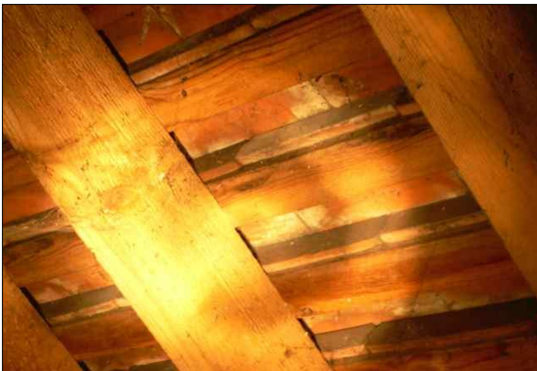
Photo15 The internal roof structure was fully accessible with the roof void. The roof tiles are hung direct onto the timber structure with no felt or roofing membrane resulting in a cold and drafty loft space.
