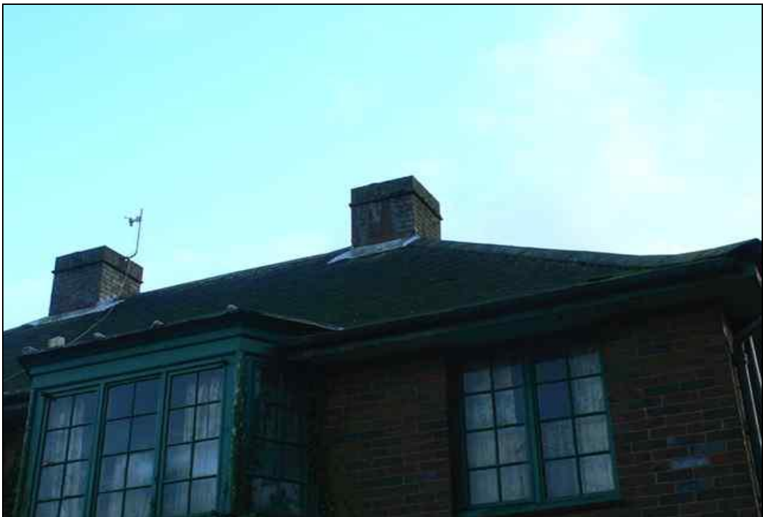
Photo 13 All upper roof surfaces were inspected for signs of bats such as dropping and staining. Particular attention was paid to roof junctions and tile gaps. No evidence of use was noted externally.
