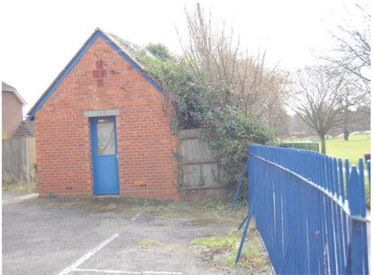
Existing store to be demolished
