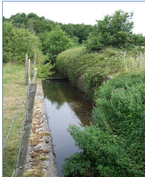
Figure 6.2 Hermitage Stream - Canalised Section
