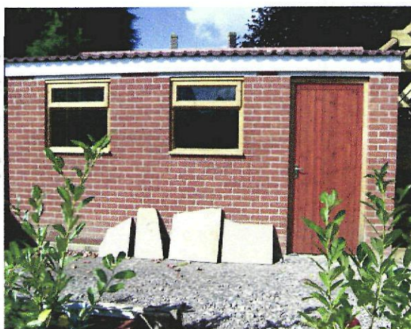
Front view of shed A South side of garden
