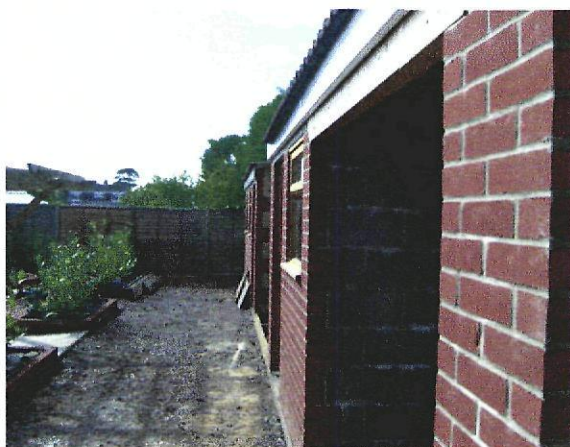
Front of sheds viewed from the North
