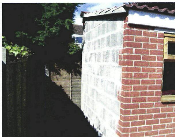
Side view of shed A Southern end of buildings
