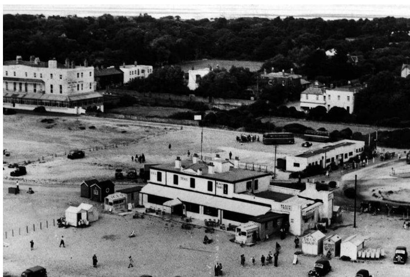
Figure 5 The Beachlands building in 1950, this remains although it has been extended to the south and the upper floor significantly remodelled.
