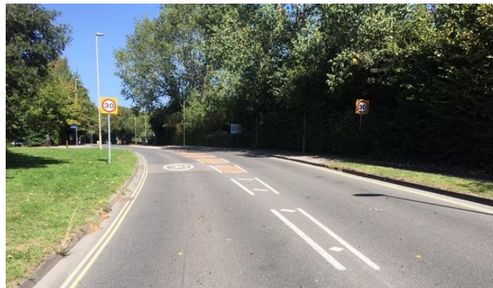
Pic 7: College Road looking northeast towards Apollo Drive and proposed location of new site access road at 30mph speed limit interface.
