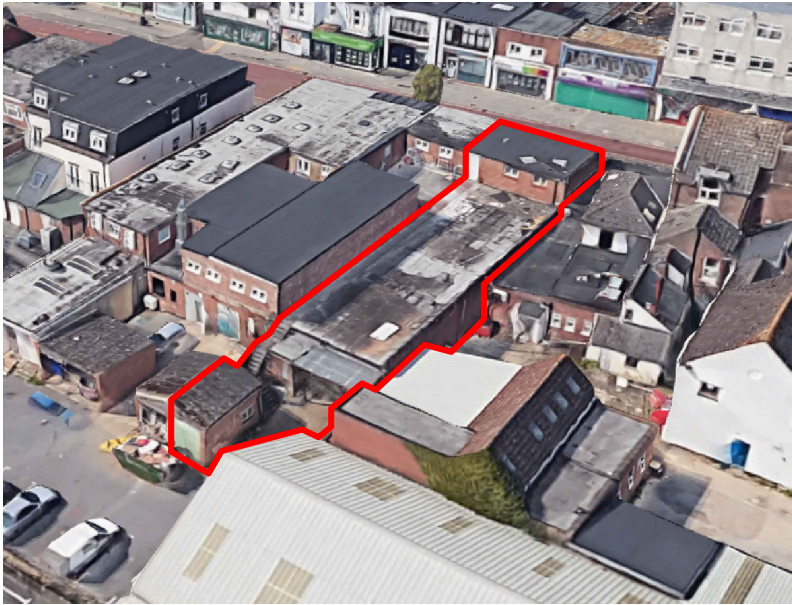
③ Aerial image of existing roofs Scale: NTS
