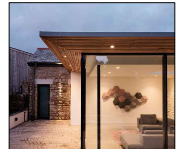
Timber cladding to eaves and end wall
