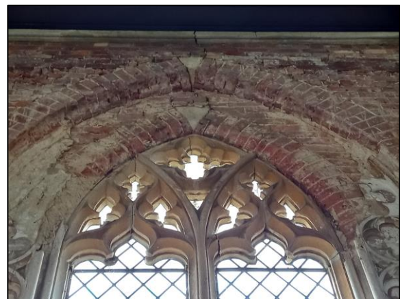
Photo 10 Brickwork above window
