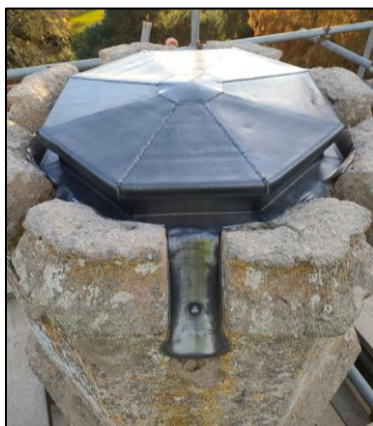
Photo 22 Chimney capping
