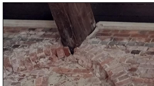
Photo 6 Main beam as it ties into wall
