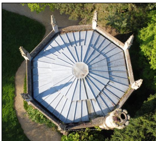
Photo 17 Drone image of roof
