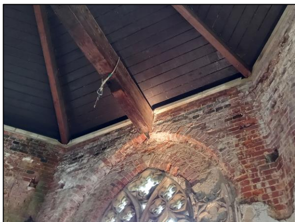
Photo 5 Main beam as it ties into wall
