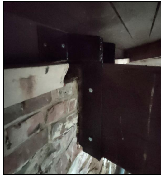
Photo 8 Bracket in place, wrapping around beam end and bolted into timber wallplate
