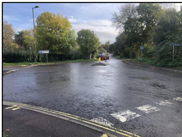
Photograph 1: Rockville Drive Conditions
