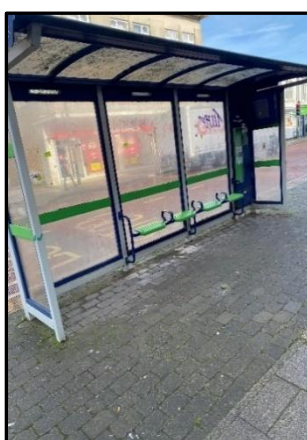
Photograph 5: Victoria Road Bus Stop (Stop E)
