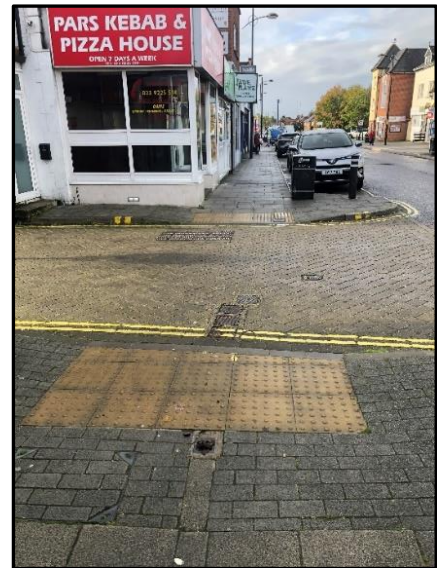
Photograph 4: Tactile Paving on Victoria Road
