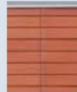
Terracotta cladding tiles as features within elevation
