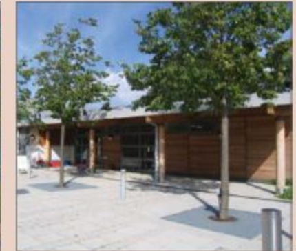
Small starter units Green Park, Reading
