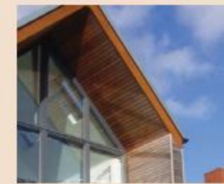
Eaves: Examples of deep eaves detail
