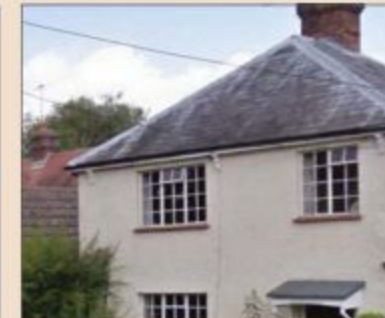
Hipped roof in Cheriton
