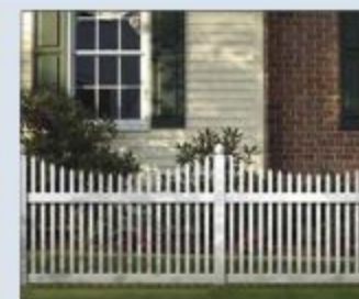
Timber fencing to frontages
