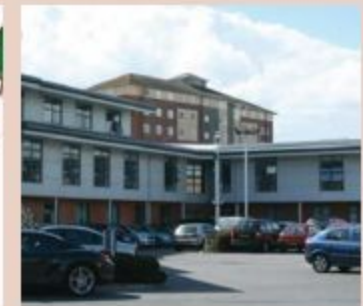
Internal parking court at Basepoint
