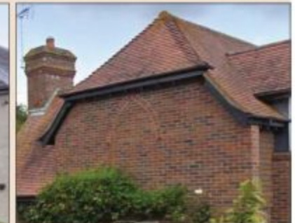
Half-Hipped roof in Cheriton
