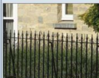
Metal railings to front property boundaries
