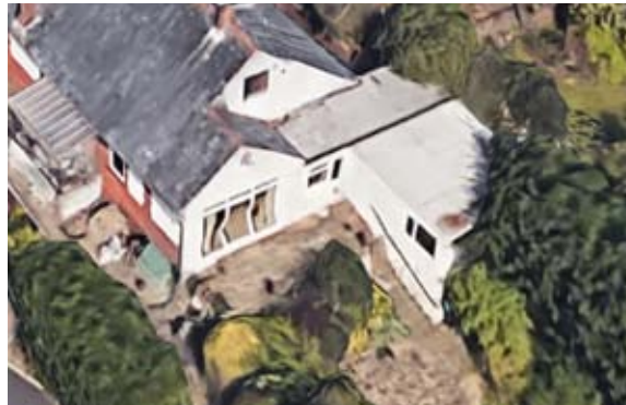
Rear / South elevation aerial view
