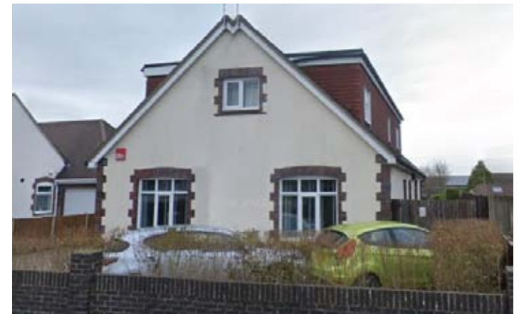
Twin dormers to 119 Stakes Road
