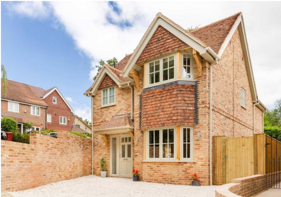
Bay window with tile hanging
