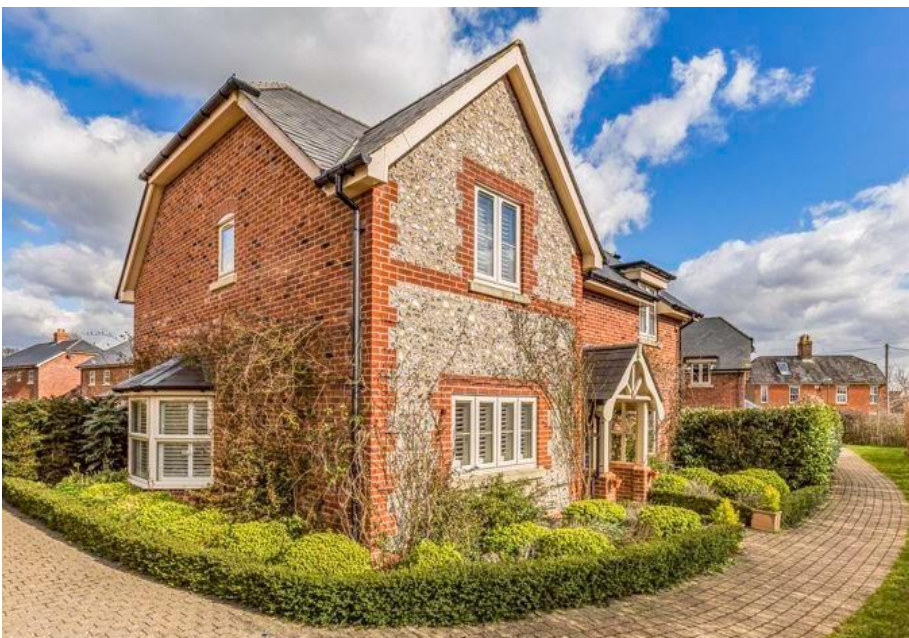
Flint gable with brick quoins at The Shire, Westbourne
