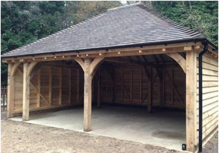
Timber framed car port with hipped roof
