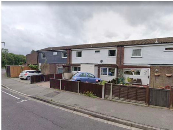
05 Two storey, wide fronted terraces Atlantis Avenue
