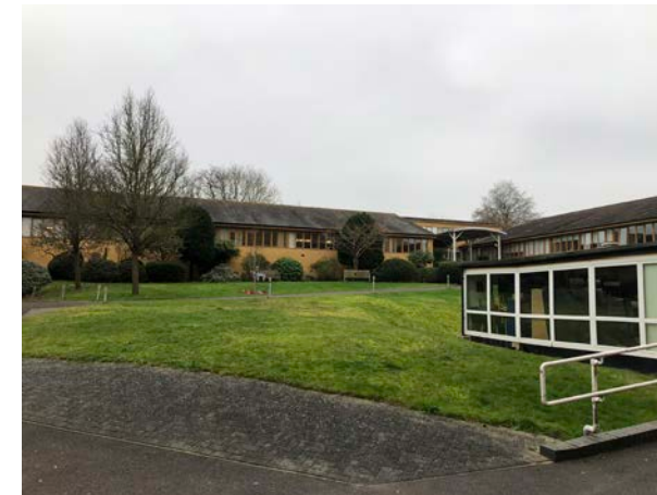
02 View from outside the site south buildings to be demolished
