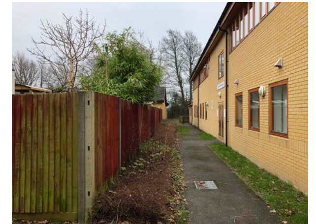
03 Fence line parallel to the existing nursery south building on the right to be demolished
