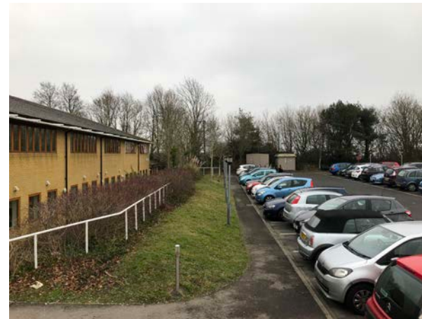
01 Edge of existing south buildings
