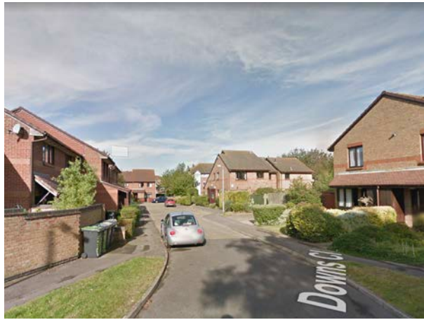
03 Brick and Clay Tile semi detached houses Downs Close
