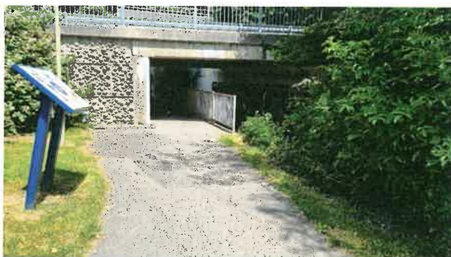
A27 Underpass viewed from south
