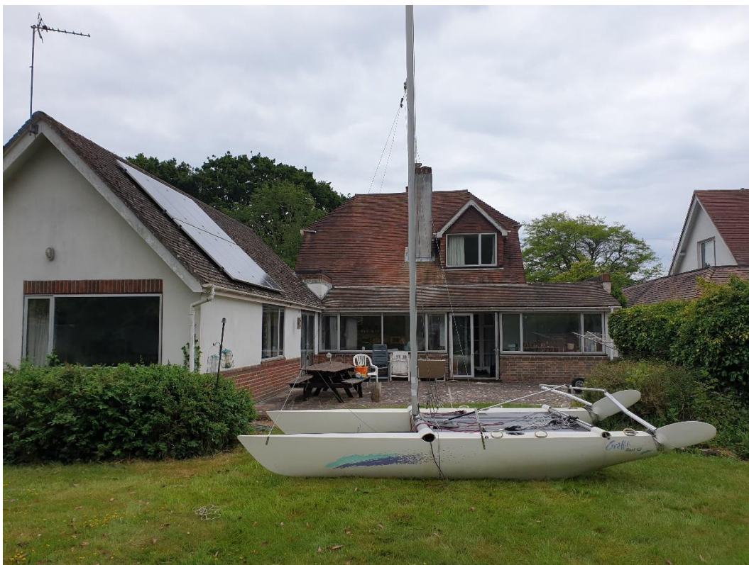
48 Sinah Lane – Rear view
