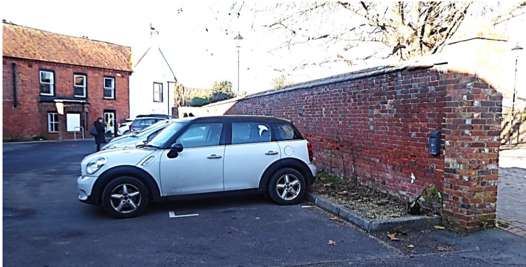
View of the inside face of the brick boundary wall
