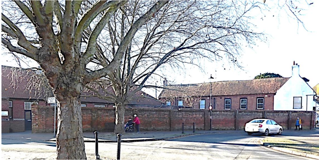
The brick boundary wall from the bottom of Fairfield Terrace; St Faith's Church House is on the right, the Church Hall is behind the wall
