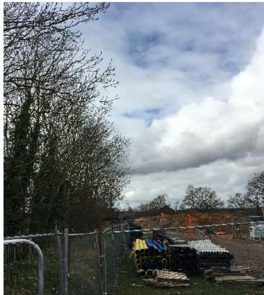
Figure 1. View looking westwards. Bartons Rd to the left.
