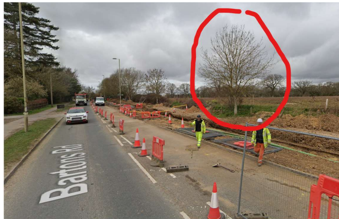
Figure 12. Google St view, Mar 2021, showing T13
