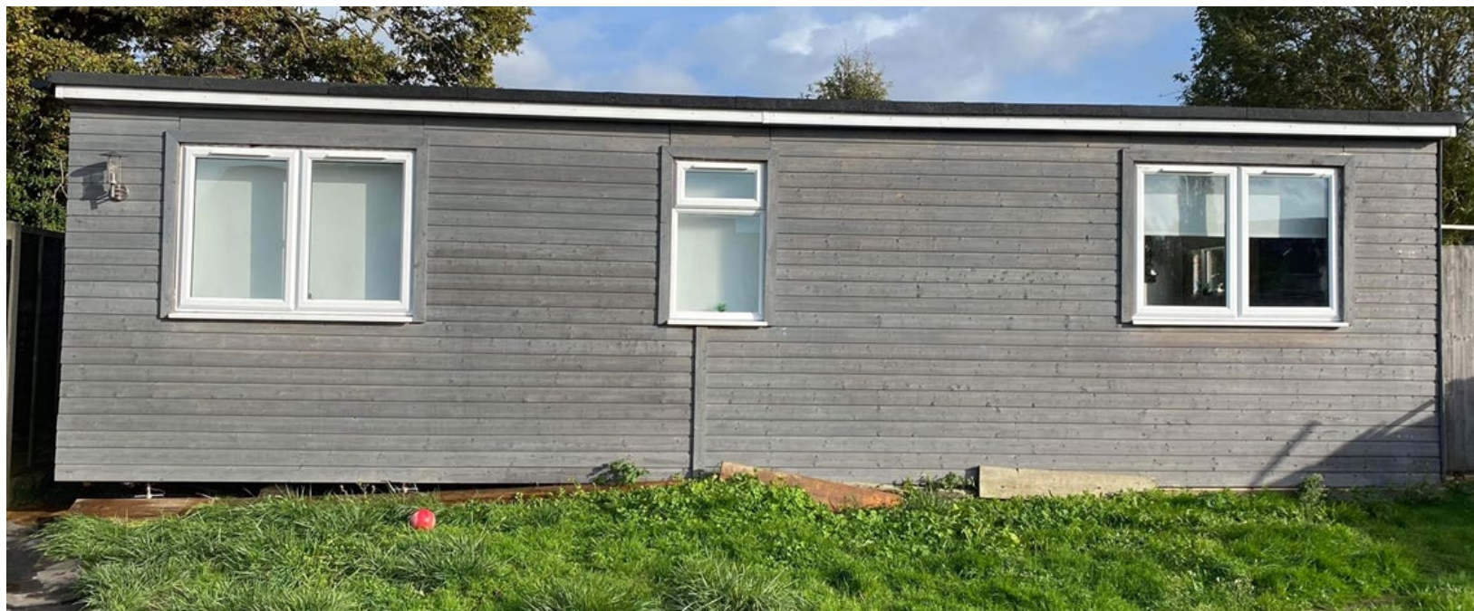
Front view of the Mobile Home facing the house at 40 Jubilee Road
