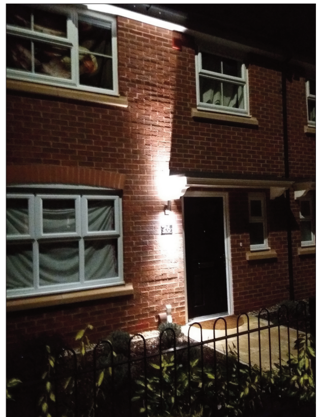
Poor porch lighting using up & down projector
