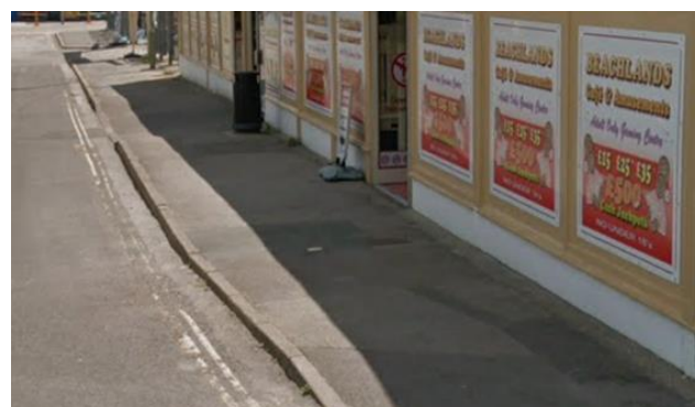
Footway flanking Sea Front
