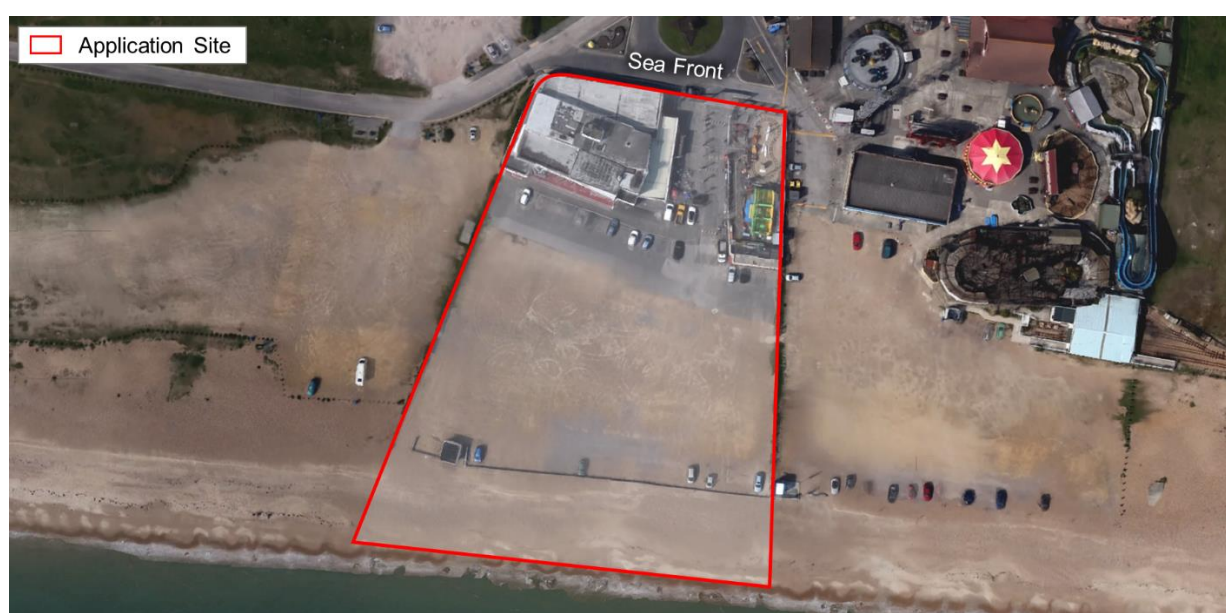
Figure 2.1: Aerial View of Application Site
