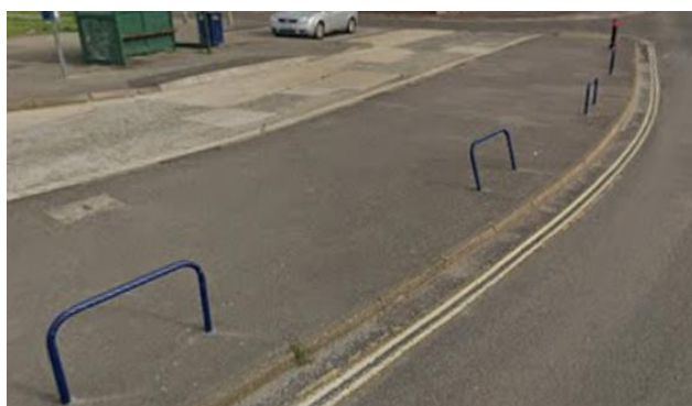
Footway to front of site
