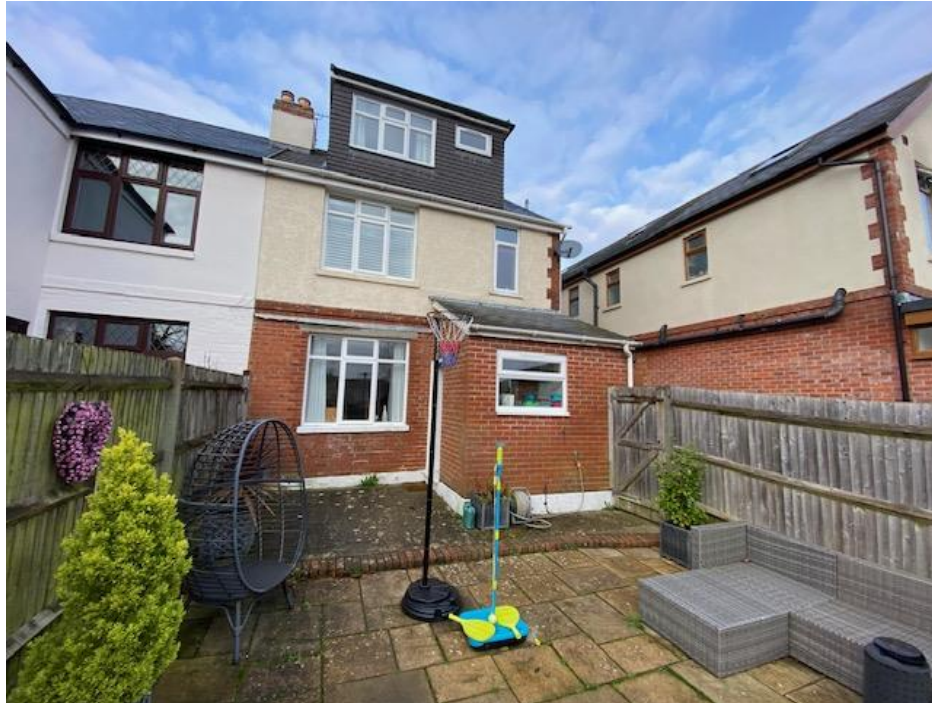
Photograph of the rear of 10 London Road showing lean-to extension
