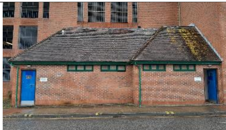
Figure 10 - View of toilet block to the east of the building.
