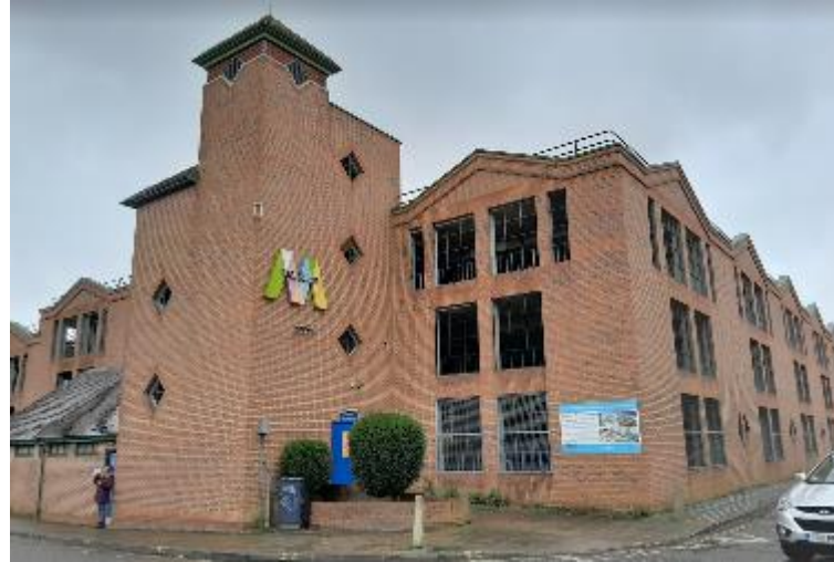
Figure 4 - View of the north and eastern faces of the building.
