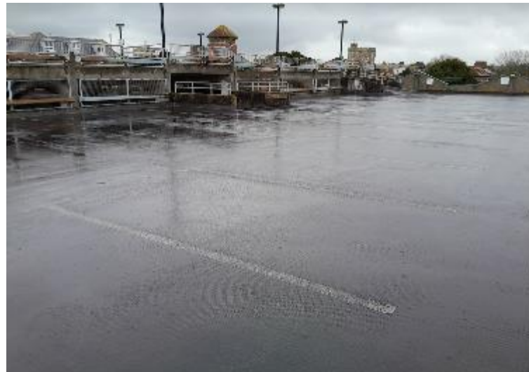
Figure 7 - View of the car park on the roof of the building.
