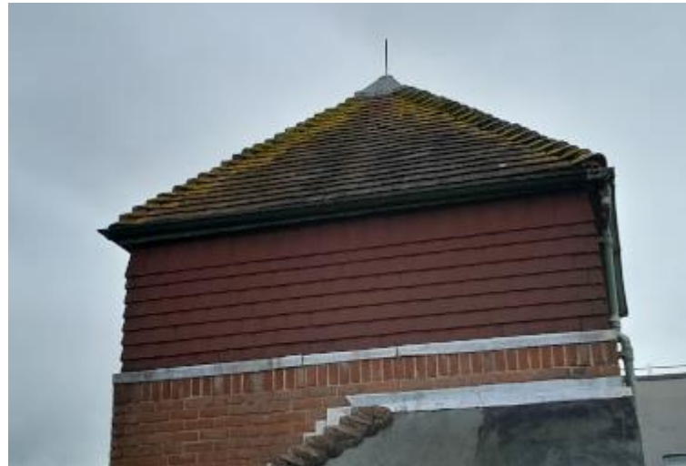
Figure 9 - View of southwestern tower showing tiled roof and hanging tiles.
