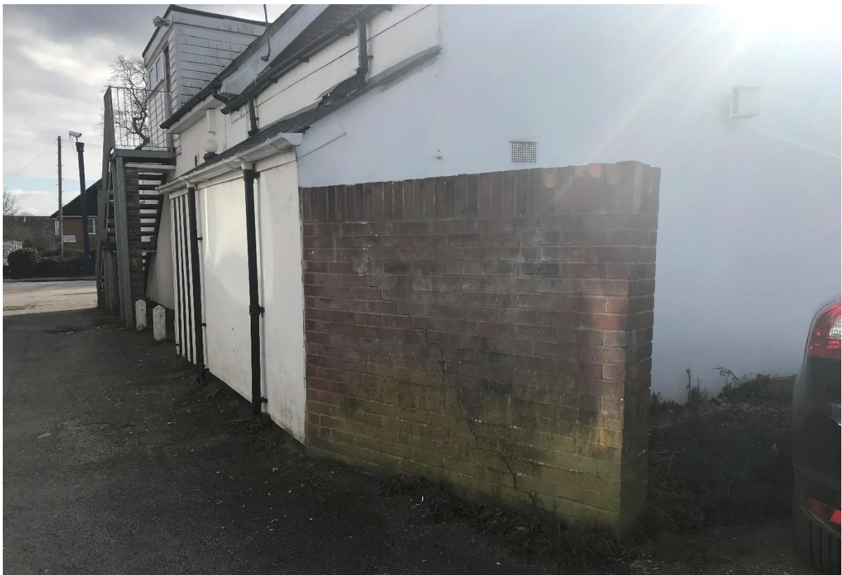
Walling at the entrance of the application site. This is to be removed as part of the development.
