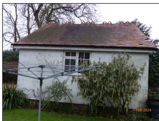
Figure 14: Northern elevation of garage.
