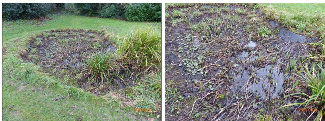
Figure 9 & 10: Mostly dry pond located in the east of the site.
