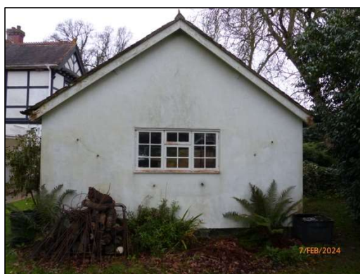
Figure 13: West facing gable of garage.
