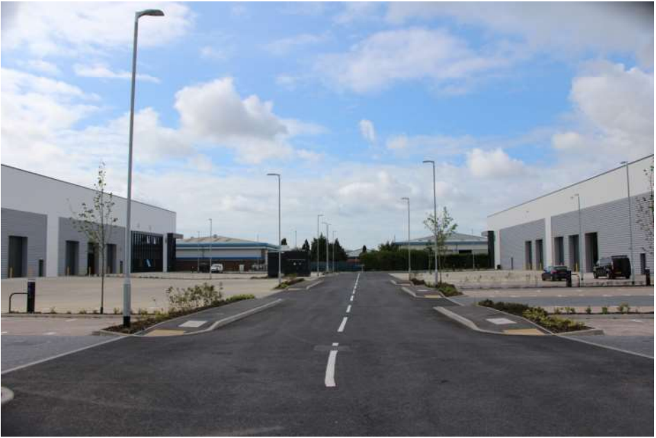
6. View from North of site showing new access road
