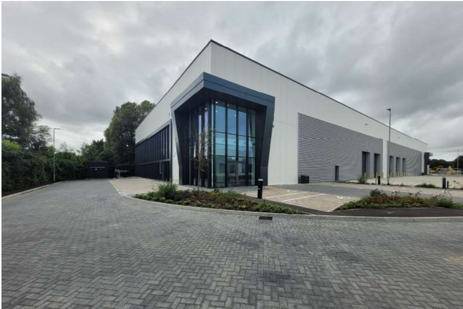
5. View from south west of site showing existing site conditions from phase 1
