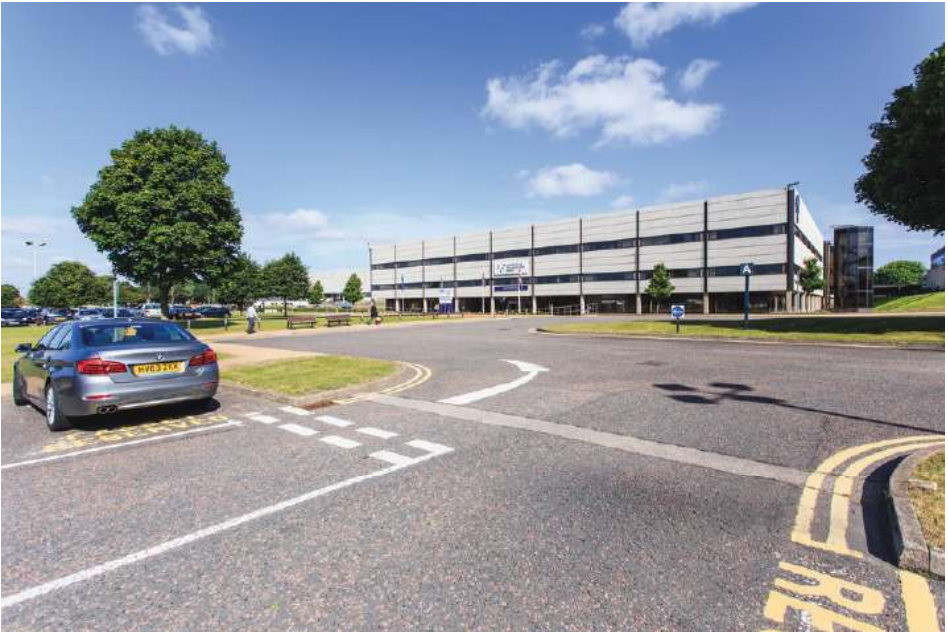
3. View from estate road toward Building 6000
