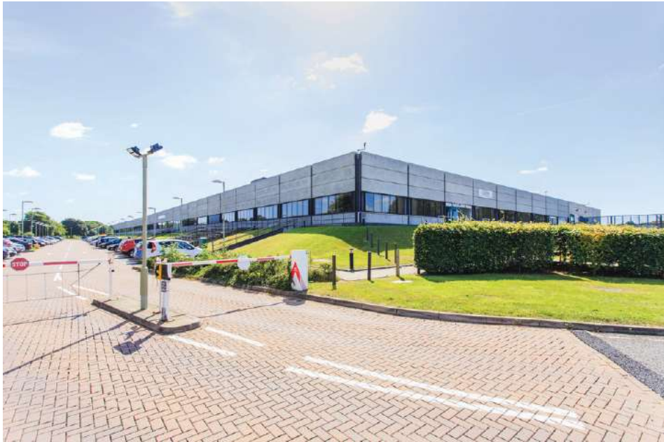
1. View from estate road toward Building 1000 and Car Park
