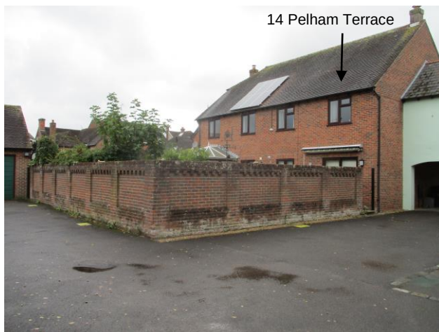
Fig.2. Rear view of the property viewed from the mews courtyard
