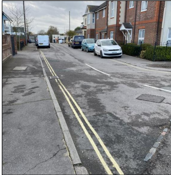
Photograph 4: Footways along Palk Road
