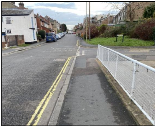
Photograph 6: Footways along West Street
