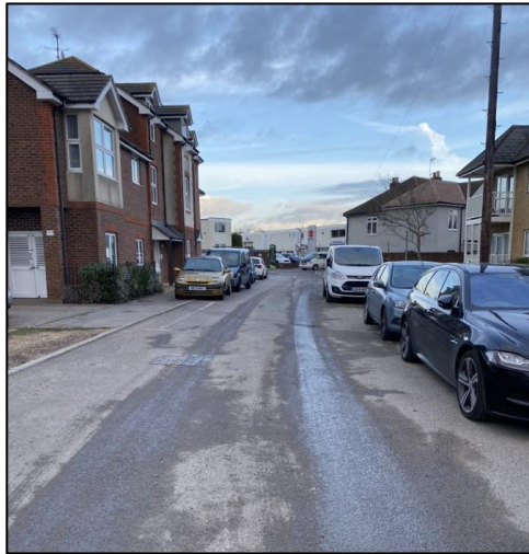
Photograph 2: Existing Conditions on Palk Road
