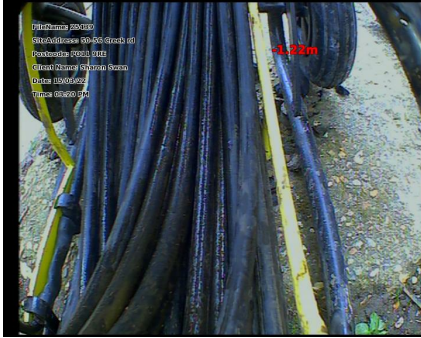
Observation [1]: Start Point: mh3
