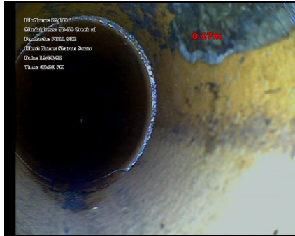
Observation [1]: Start Point: mh3
