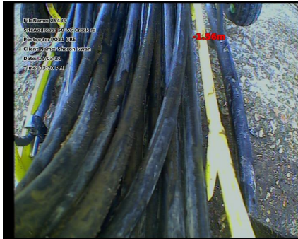
Observation [1]: Start Point: mh2
