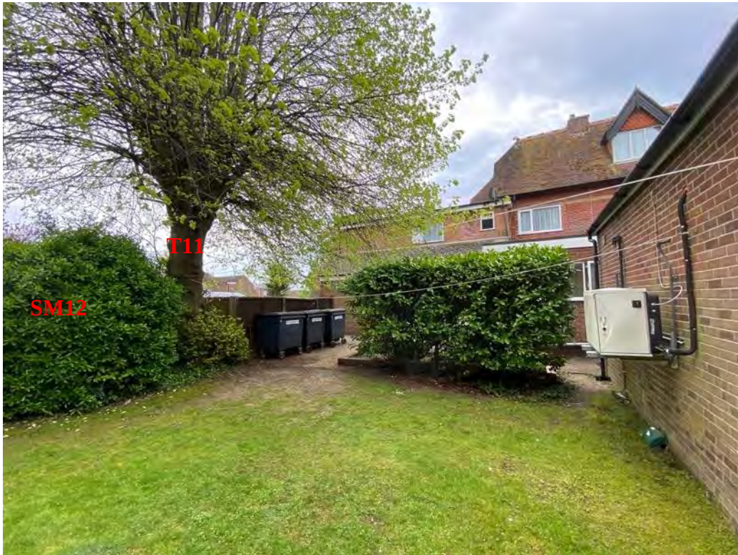
Photoview 7: View south at T11.
