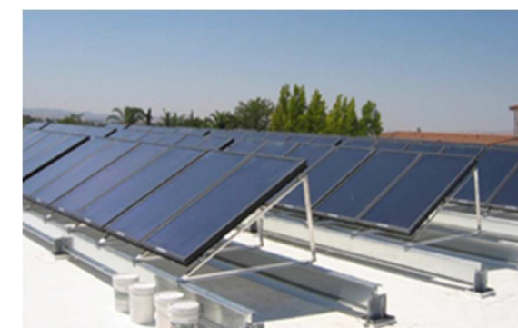
Picture 2—Frame mounted PV on flat roof
