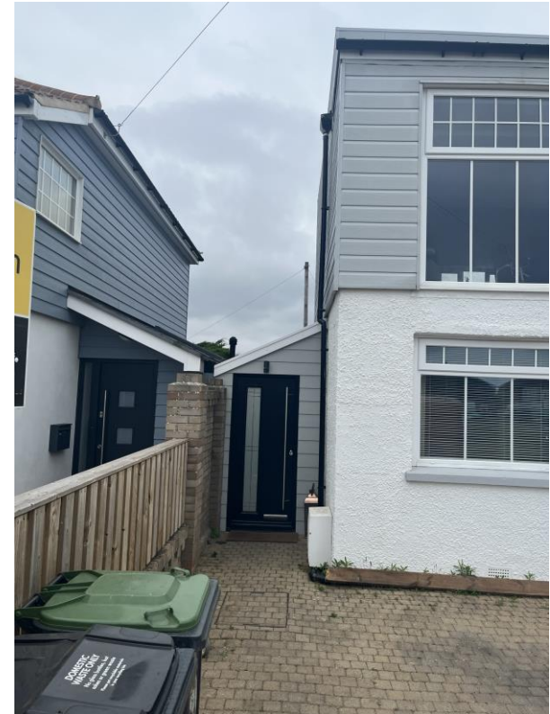
Existing front access
