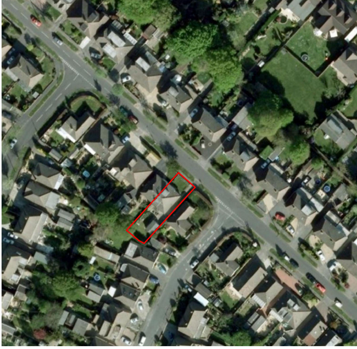
AERIAL VIEW OF CHERRY TREE AVENUE AND SURROUNDING ROADS (No.29 outlined in red)
