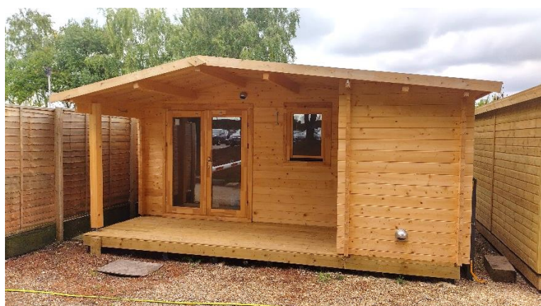
Photo 1 Existing 'Maidstone' wooden outbuilding (5.3m x 4.5m) used as office.
