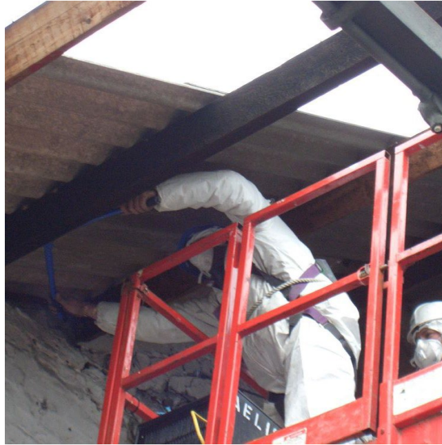
Bonded Asbestos Roof Sheeting Removal Works
