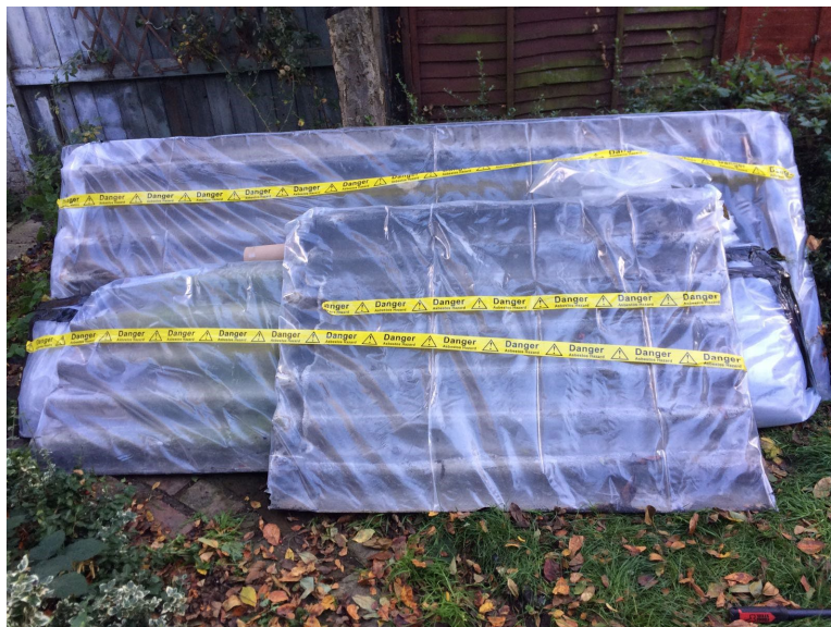
Bonded Asbestos Roof Sheets Removed
