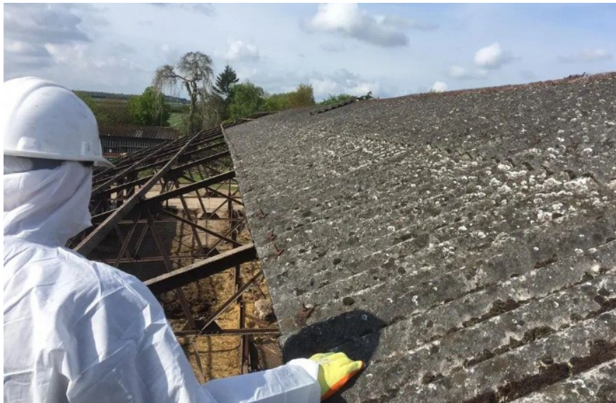
Bonded Asbestos Roof Sheets Removed
