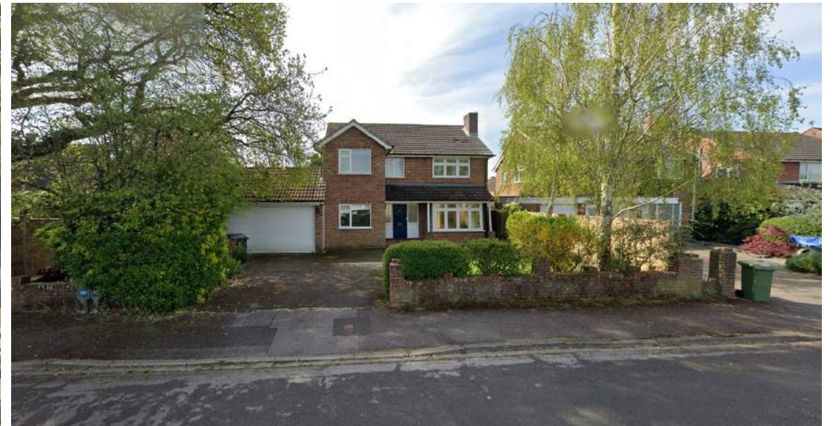
Above / Views of front of no.50 from Woodlands Avenue.
