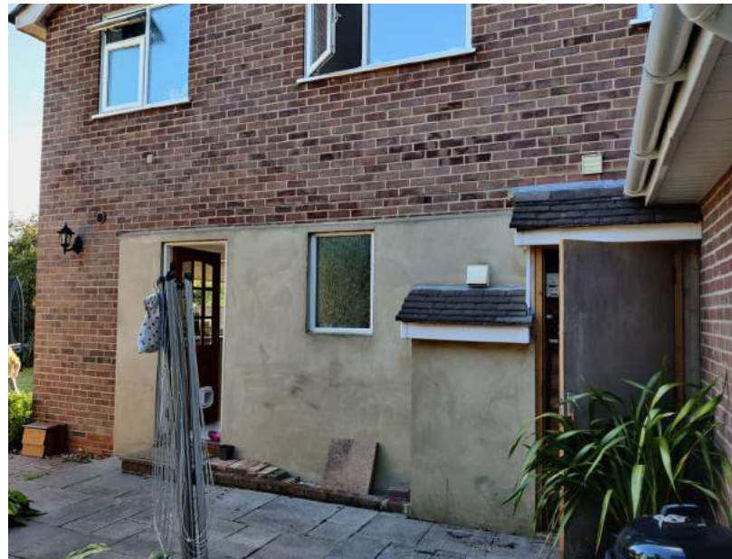
Above / View from behind existing double garage.
