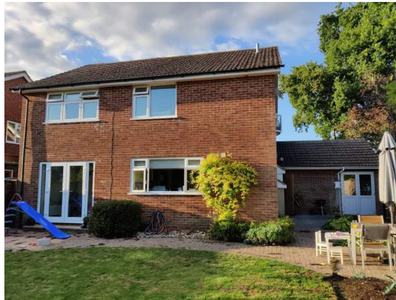
Above / View of rear of no.50 Woodlands Avenue.
