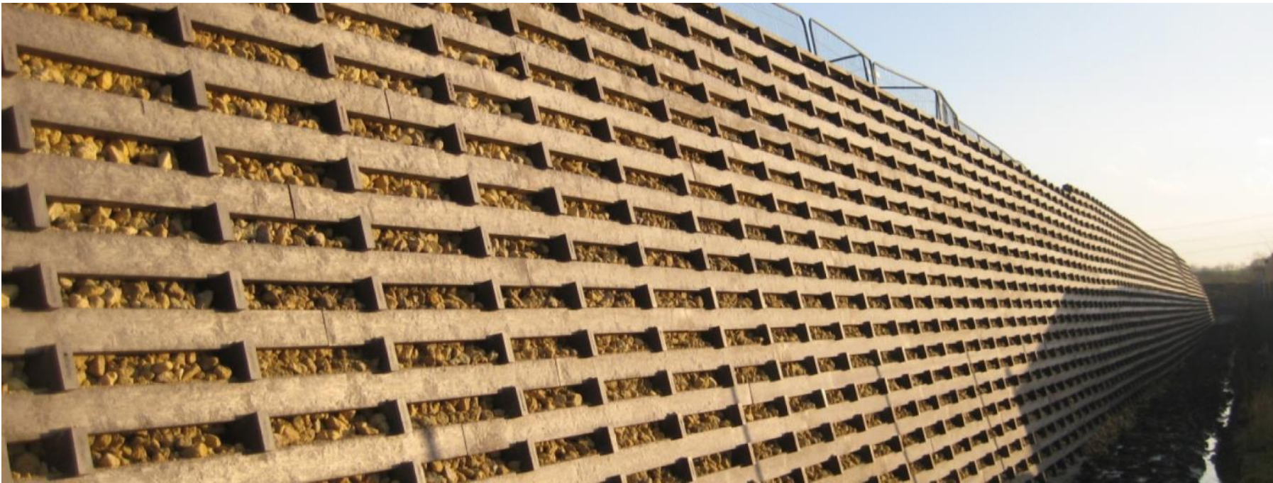
Cribb retaining wall
