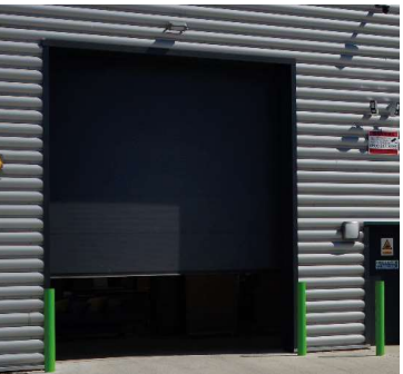
LOADING DOOR & STEEL BOLLARDS
