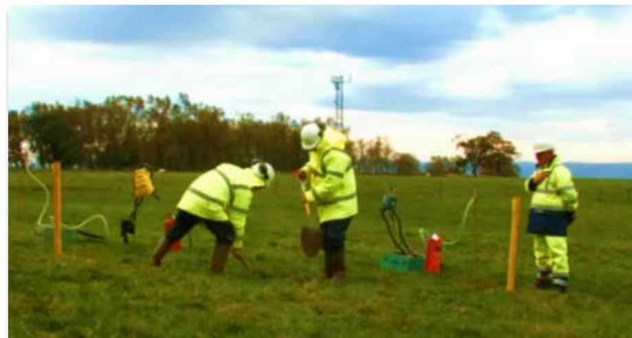
Figure 4. Hand Excavated Trial Hole
