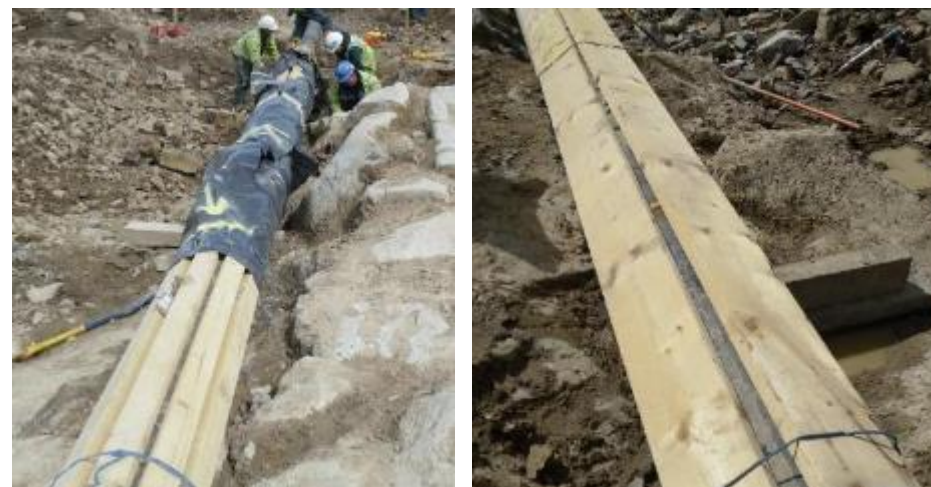
Figure 14. Protective cladding applied to pipeline
