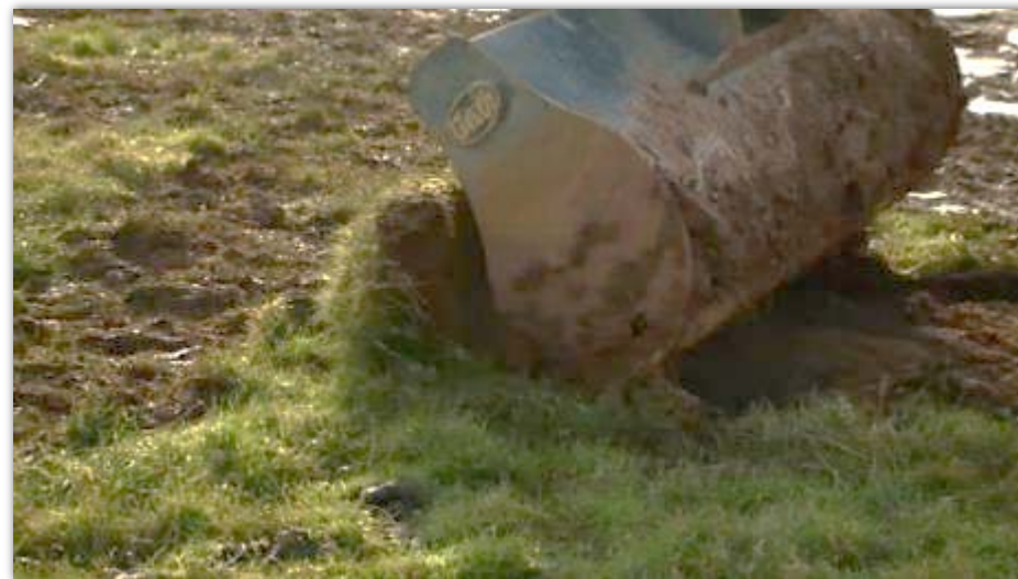
Figure 12. Top Soil Stripping
