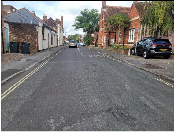
Photograph 4: Existing conditions along Town Hall Road
