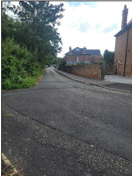
Photograph 6: Existing conditions along Grove Road
