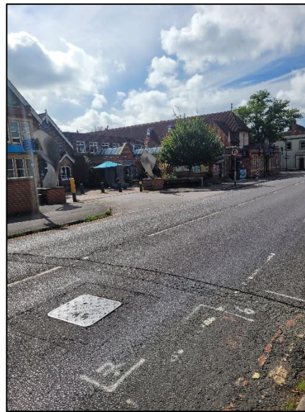
Photograph 3: Existing conditions on East Street
